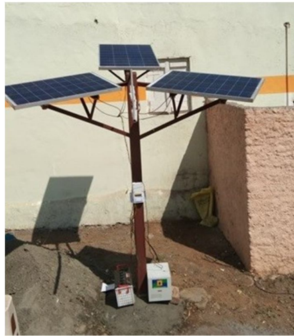
Figure. 2. Installation of 1kw Solar Tree
